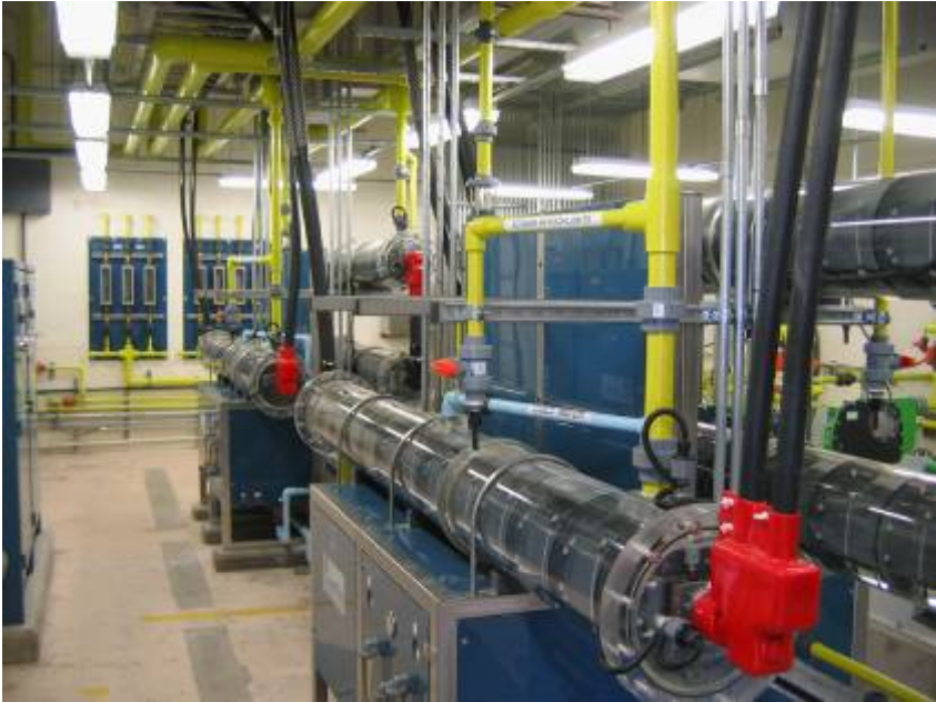
The ClorTec™ CT Series Sodium Hypochlorite Generating System from Severn Trent Services
