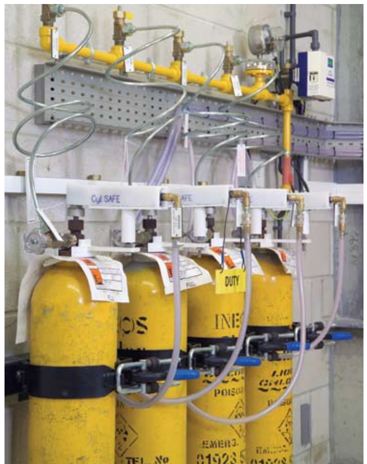
Cyl-SAFE Automatic Shutdown System
