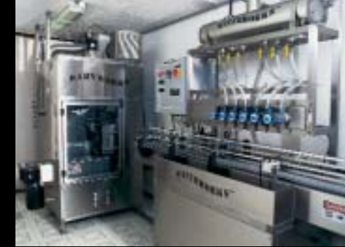
Custom Electrical, Plumbing, Insulation Installation
