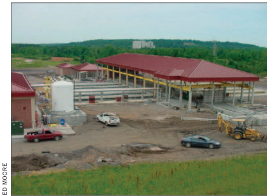
The Village Creek stormwater filtration plant nearing completion. The $300 million facility can handle up to 360 mgd (1.4 million m 3 /d) of wet weather flow for 4 hours.
