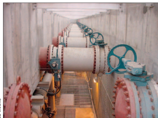
Village Creek's filter influent piping and valves conduct plant influent from a concrete influent channel to the facility's filters.
